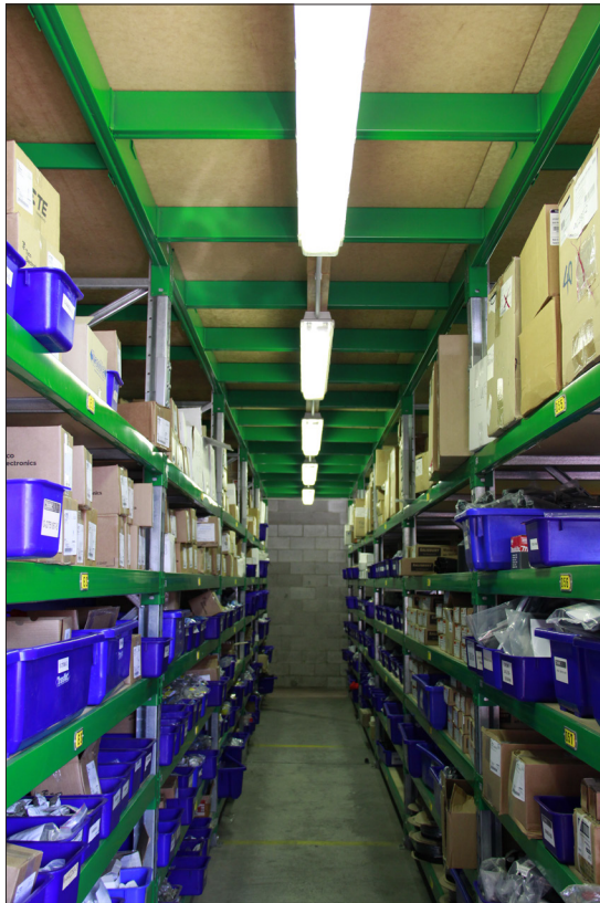
Before: Low level picking isle illuminated by fluorescent tubes, poor light spread.
