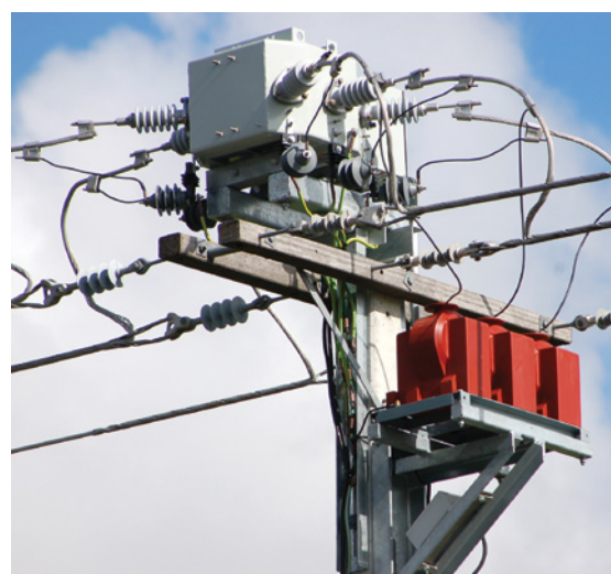
Pole Top Mounted Rotary Puffer Switch
